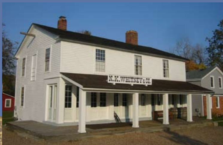
The Newell K. Whitney's store was a gathering place and general store for residents of 1830s Kirtland. Today the store is maintained and preserved by the Church of Jesus Christ of Latter-day Saints.
